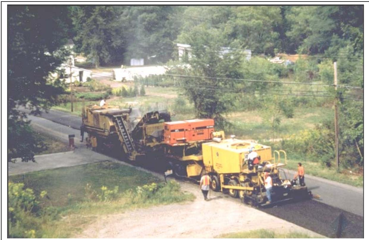
**Figure 12. Cold In Placed Recycling Method of Flexible Pavements**
